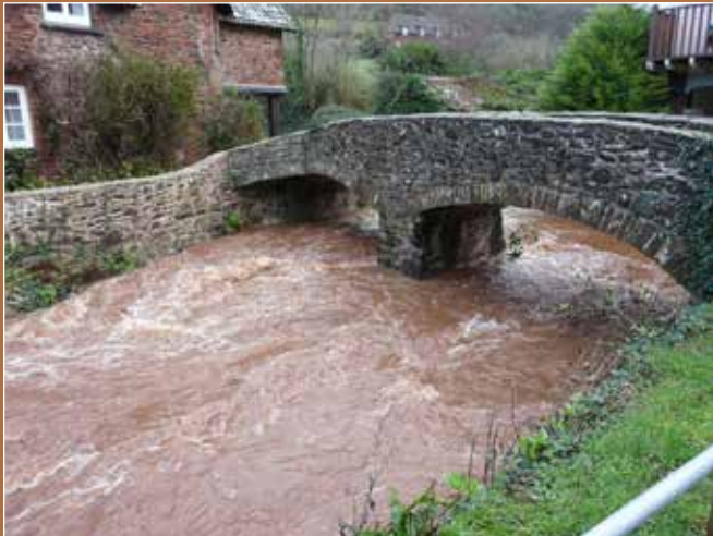
Sediment laden floodwaters in Allerford.
