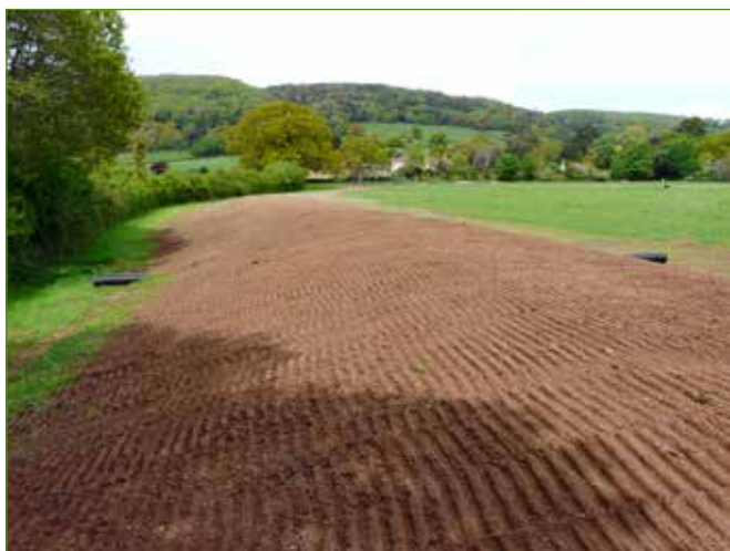
Left to right: Shallow earthen flood storage bunds on Aller floodplain; Aller leaky sluice; Aller river level gauge; and Raingauge station.
